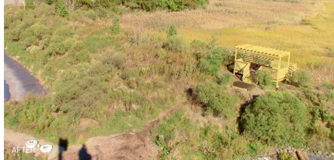
Wetland restoration, Port Newark, US
