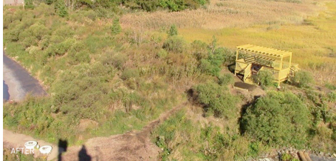
Wetland restoration, Port Newark, US
